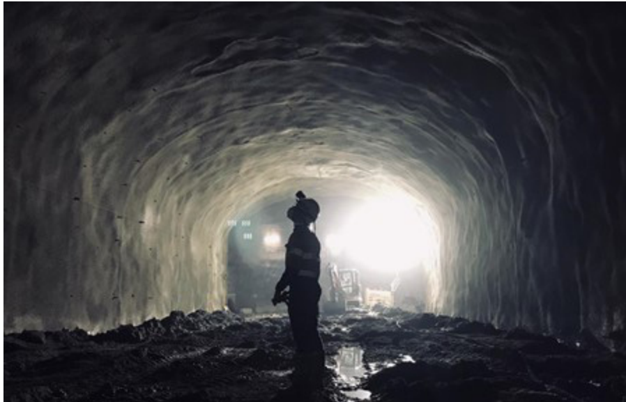
Second Place: A site engineer inspects a tunnel in the calm before the next shift, Sydney, Australia. Photo by Eva Grasso, Australia.
