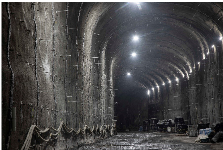
First Place: Tunnel "spikes" - Depth pins prior to the secondary shotcrete lining. Photo by Tom Roper, Australia.
