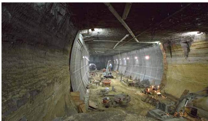
Figure 2. LRT station under construction.
