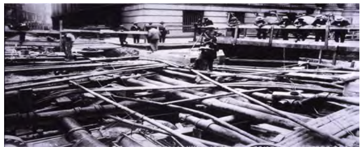
Figure 11. Subsurface facilities revealed during excavation, Wall Street, New York (ca. 1917). 61
