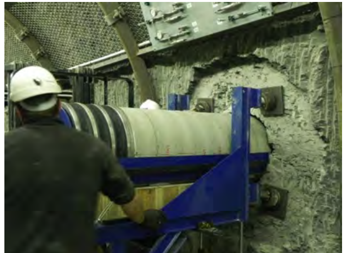
Above: Figure 1. Work on the in situ experimental studies at the Tournemire site in France.
