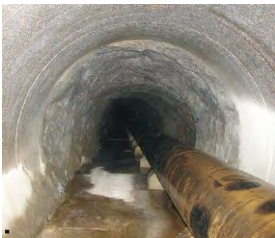
Left: Figure 5. Bedrichov water tunnel in the Czech Republic.
