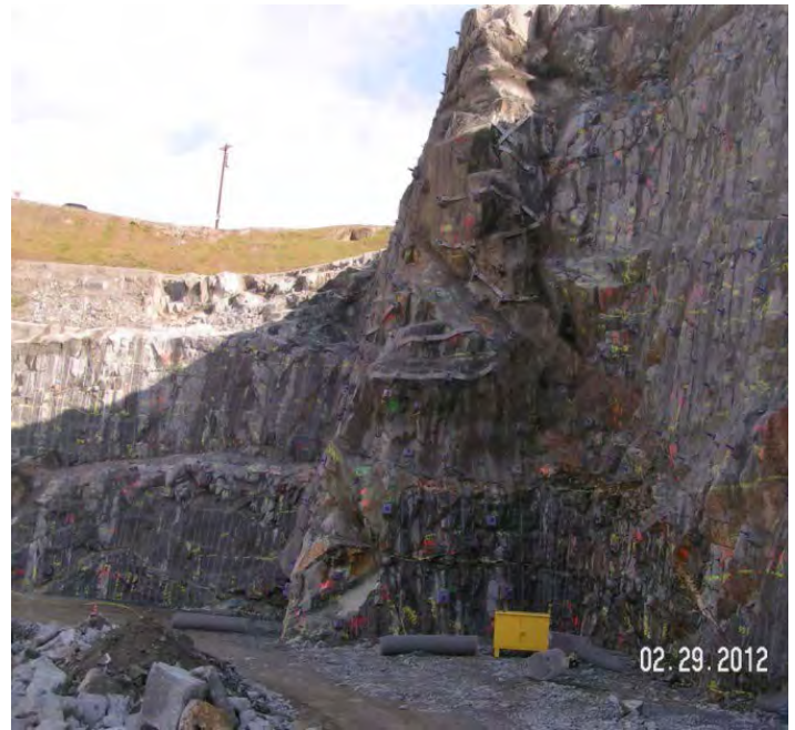
Figure 3. Emergency Spillway Control Structure, Folsom Reservoir (California)
