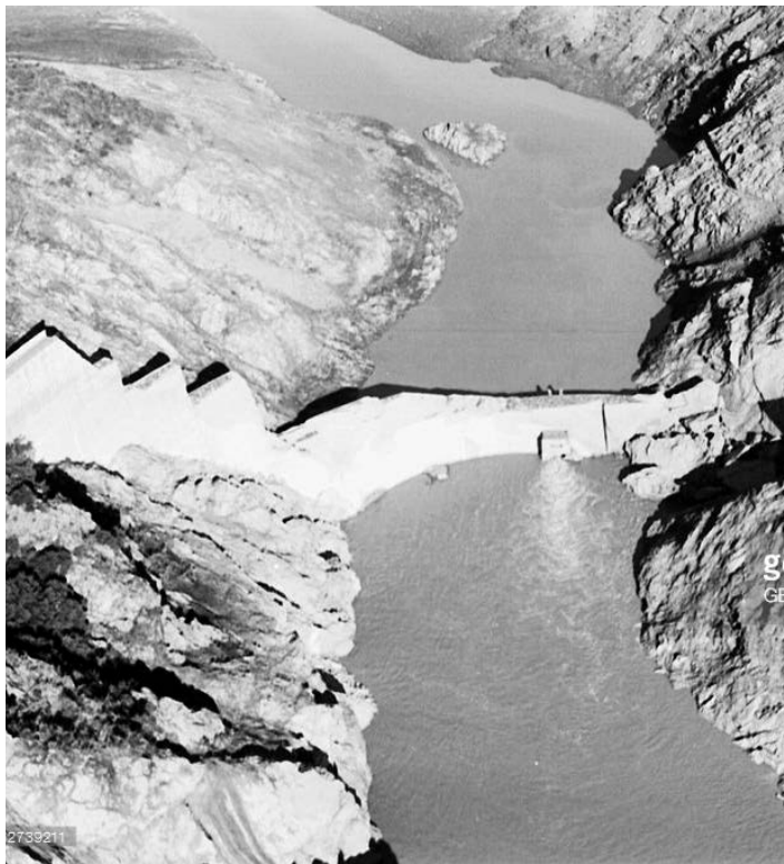
Figure 1. The remains of Malpasset Dam (France).
