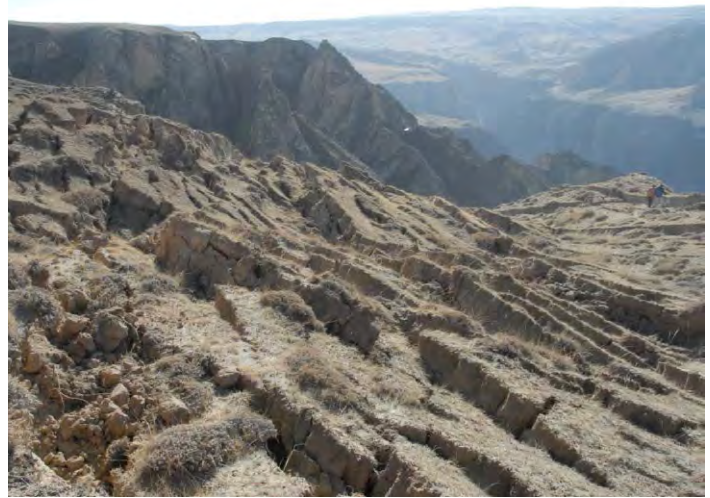
Figure 5. The surface of the enormous toppling failure immediately downstream to the high Laxiwa Dam (China).
