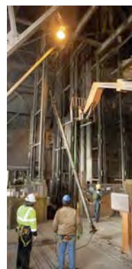
Figure 7: Equipment that is too large to fit in the cage must be slung underneath the cage
