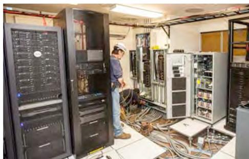
*Figure 8: Jason Rath, Facilities Tech in black shirt, and Industrial Electrician Warren Weller install cable for new electrical services in the server room. Note the open cabinet that houses the UPS.*
