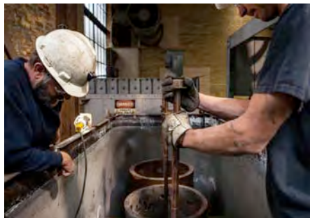
Figure 5: Facilities Technicians Kevin Ehnes and Chris Huber install electrodes into the clay pots in the slip regulator tank
