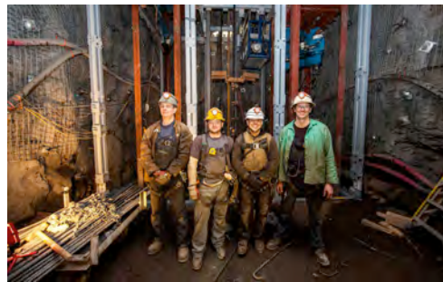
Figure 9: Infrastructure Techs Jerry Hinker, Loren Larsen, Derek Lucero, and Joe Nonnast at the 300 Level, with the vertical steel (gray) in place. Red structures are work decks
