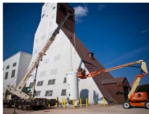
*Figure 4: Facilities Tech Kevin Ehnes (in the basket) operates a lift to reach the straps used to hoist the new liquid nitrogen bulk tank into place*
