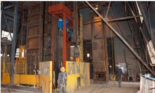
*Figure 5: Infrastructure techs Loren Larsen, Chris Huber, and Jeff Essink helped remove the north skip from the Ross Shaft. The skip is the tall brown device at the back of the photo. Larson inspects the work deck (red) in the cage compartment of the shaft. The new crane (blue) is attached to the top of the work deck*
