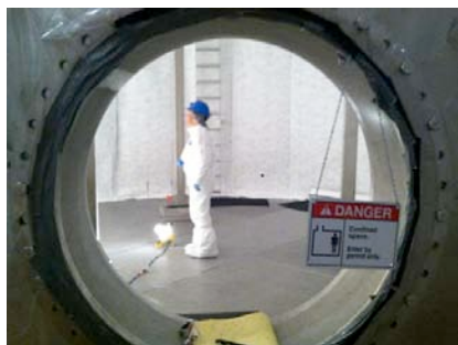
Figure 2: Mia Ihm, underground in the water tank during the PMT installation
