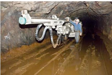
*Figure 4: September 2009 photo at the 4850 Level - Sanford Lab Underground Operations Foreman Jack Stratton behind the 20-foot boom of the jumbo drill. Note the watery floor!*
