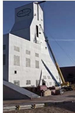
*Figure 9: Heavy Constructors Inc. contractors open a window on the south side of the Yates Shaft headframe*
