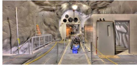
*Figure 8: The new top floor of the Davis Cavern. Room at right will be the control room for the LUX dark-matter detector. Wide doorway in the center leads to the Transition Area where the MAJORANA DEMONSTRATOR experiment will be installed*
