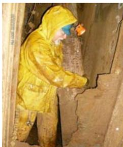
Figure 6: Infrastructure Tech Larry Cornella removes wood lacing from the Ross Shaft near the 3650 Level
