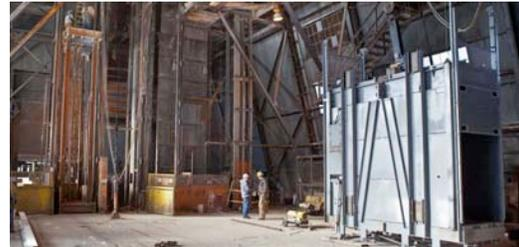
Figure 7: New service cage ready for installation. The old work deck is still in the shaft.
