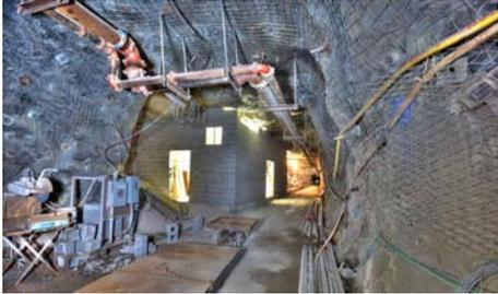
Figure 5: Block wall in the chiller cutout on the 4850 Level
