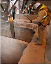
*Figure 9: Project Safety Officer Steve Sandman of Heavy Constructors Inc. oversees the concrete pour for the south footing of the rope-dog tower*
