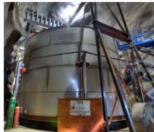
Figure 3: The LUX water tank awaits one more row of stainless steel plates before being welded together
