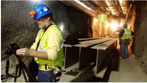
Figure 5: At the Transition Cavern: Computer Science Professor Steve Graham of Dakota State University is helping to build a virtual Sanford Lab. The I beams behind him will eventually be moved to the Davis Cavern
