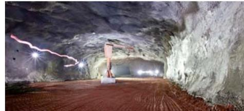
Figure 12: Shotcreted walls and ceiling in Transition Cavern with engineered fill on the floor
