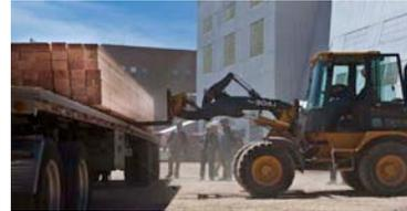
Figure 10: Infrastructure Tech Kevin Ehnes operates the loader as new shaft guides are installed at the Yates Shaft to provide better access to the 4850 Level
