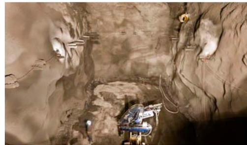
*Figure 7: View of Davis Cavity from Transition Cavity as crew member prepares to apply layer of shotcrete*
