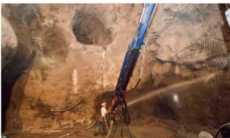
*Figure 6: Contractor wets down the Davis Cavity walls in preparation for applying shotcrete*
