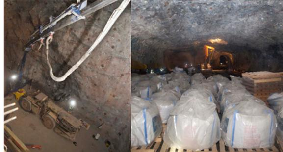
*Figure 10: (left) Robotic arm in Davis cavern can be operated from the ground to apply shotcrete in hard-to-reach places; (right) Bags of shotcrete with hoist in background*
