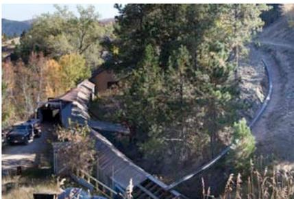
*Figure 9: Pipeline is buried: the new trench will redirect water from underground to the Mill Reservoir. A second new line in the trench will transport Grizzly Gulch water to the reservoir. The new system will provide a more stable, reliable flow of water to the Sanford Lab treatment plant.*
