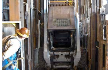
Figure 5: Rick Tinnell of CAI Construction (secured by a fall protection harness) observes Bobcat delivery
