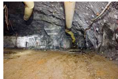
Figure 2: View from the entrance of the Transition Cavern
